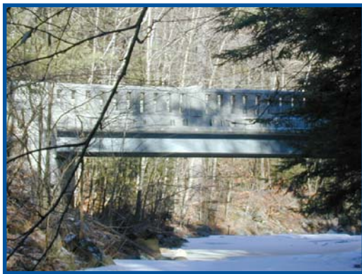
HEATH RD. BRIDGE, COLRAIN, MA
