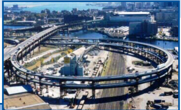
Inverset™ units were used successfully on this Central Artery North Area (CANA) project in Boston – longitudinally, as simple spans and transversely as decking units.
