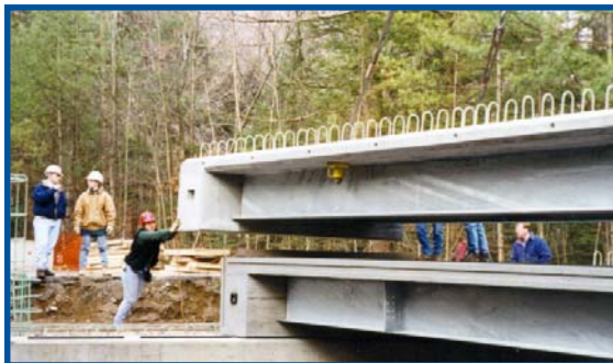
HEATH RD. BRIDGE, COLRAIN, MA
