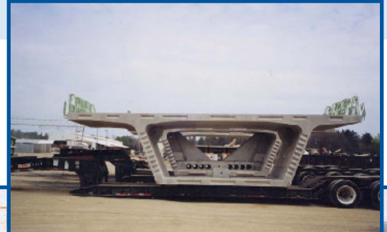
Segments on the trailer and ready for shipment to the Brooklyn-Queens (NY) Expressway Connector Ramp Project.
