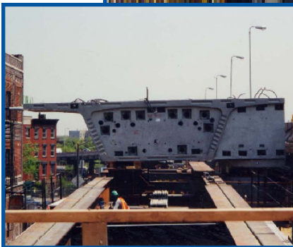
Pier No. 2 Segment looking East.
