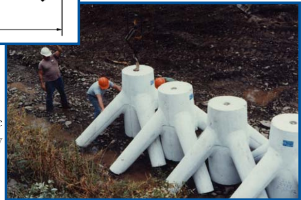
RIGHT: Installing Sta-Pod™: the bottom legs interlock to securely protect the area from scour.
