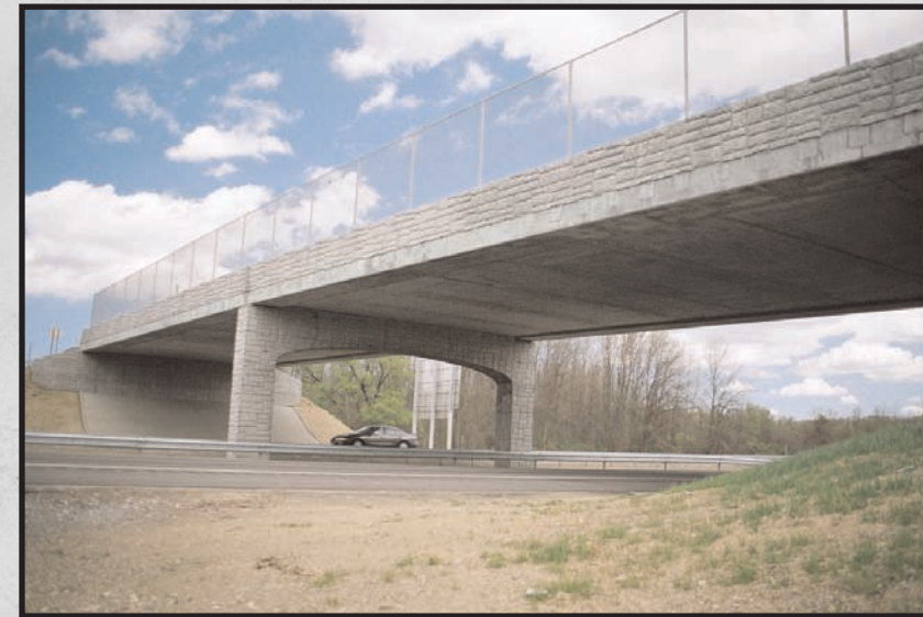
Hook Road over The New York State Thruway, Rochester, NY. Form liner finish on edge girders matches abutments and the pier.
