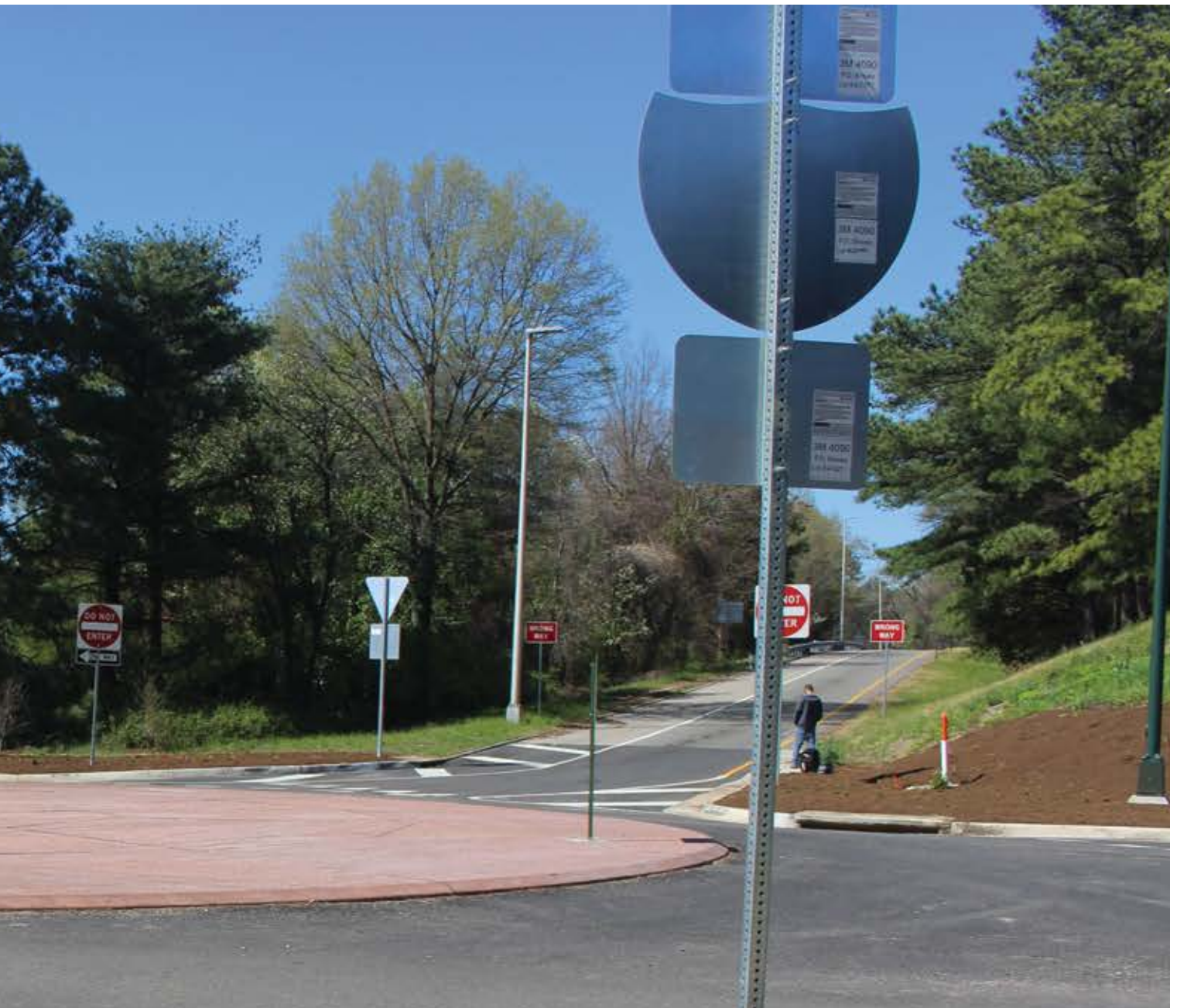
New York-based The Fort Miller Co. worked with the Virginia Department of Transportation to design and install the first-ever precast concrete roundabout in the United States.
